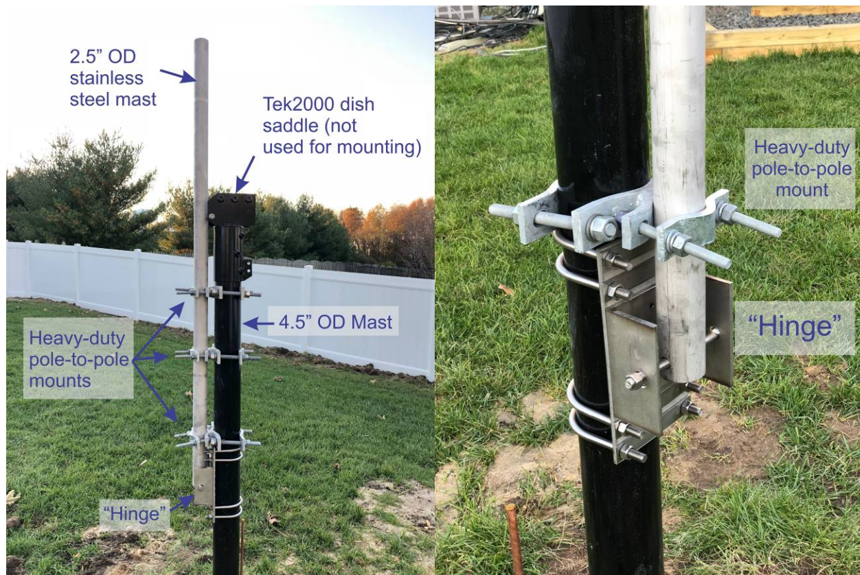
Figure 4 - The actual mast onto which the rotator is mounted is a 6'-long, 2.5" OD thick-wall stainless steel tube held by heavy-duty pole-to-pole mounts. A tilting bracket is used to allow the rotator and hub to be assembled and at floor level. The hinge bears no load once the mast is secured by the pole-to-pole mounts.
